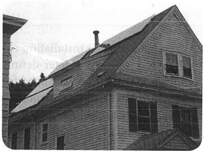
These solar panels low profile and location make them unobtrusive even though they are visible from the public right of way. Photo by Paul Trudeau
